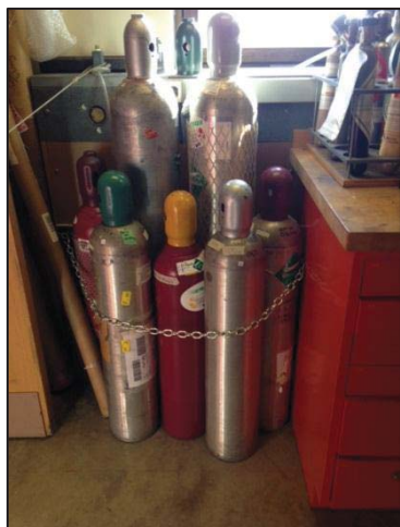
Figure 5.3 – Not In-Use Cylinders
